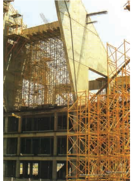
Istanbul Olympic Stadium mega-structure rack beam shorings, MKH 150 system
