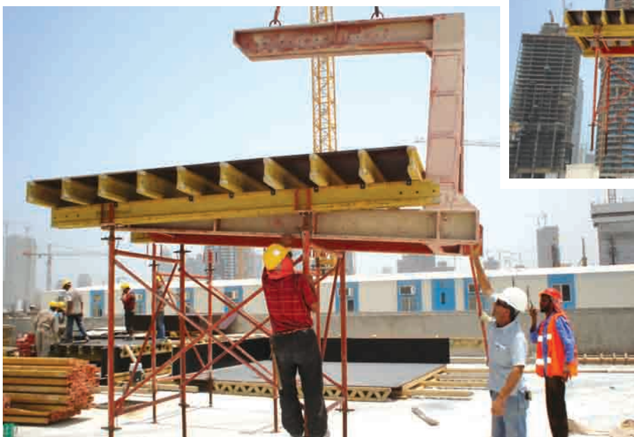
MKH 150 tables flying at Dubai sky's with table lifting fork.
