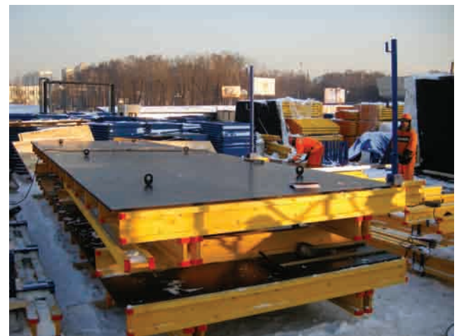
Eye-bolts, ready lifting the table panels
